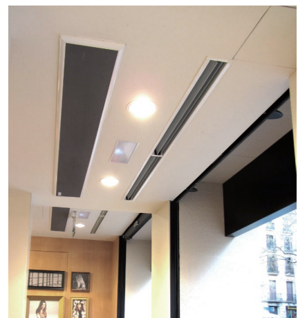
Windbox Invisible Installation with false ceiling kit
