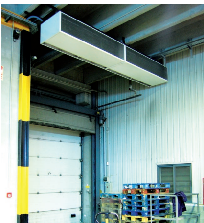
Windbox L Multiple installation in an industrial door
